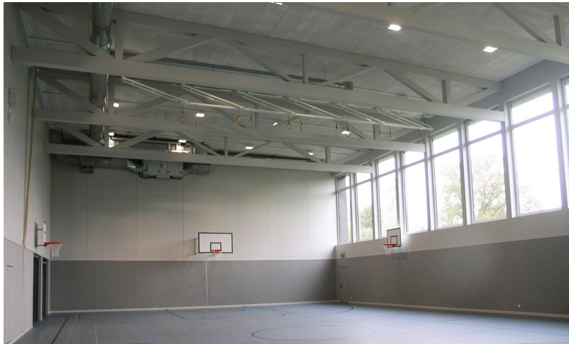
Temporary prefabricated construction
