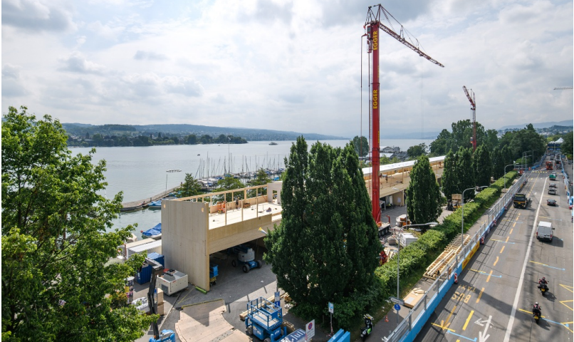
Building a temporary pit lane
