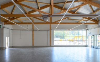
Exposed timbers inside Generous sales rooms
