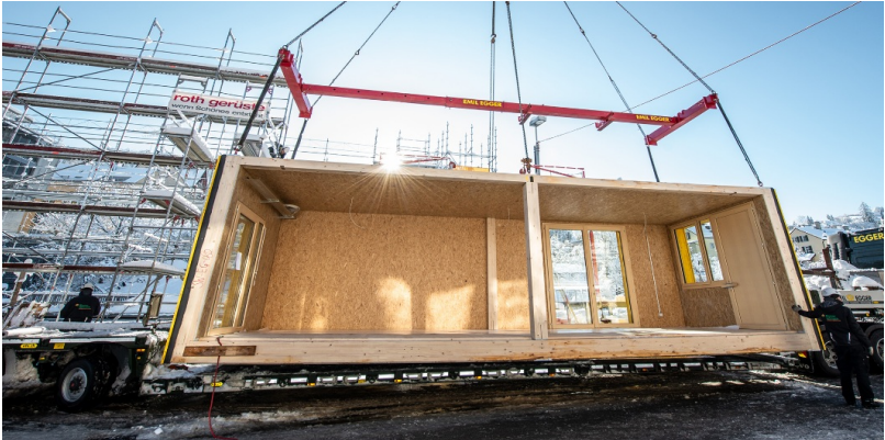
The Lattich building in St Gallen is made up of 48 modules
