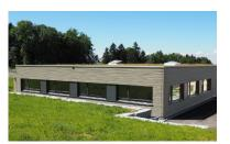
The second floor of the office building and the roof are a wood element construction.
